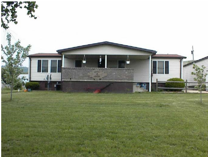
Figure 3.1 Pennsylvania double-wide trailer
