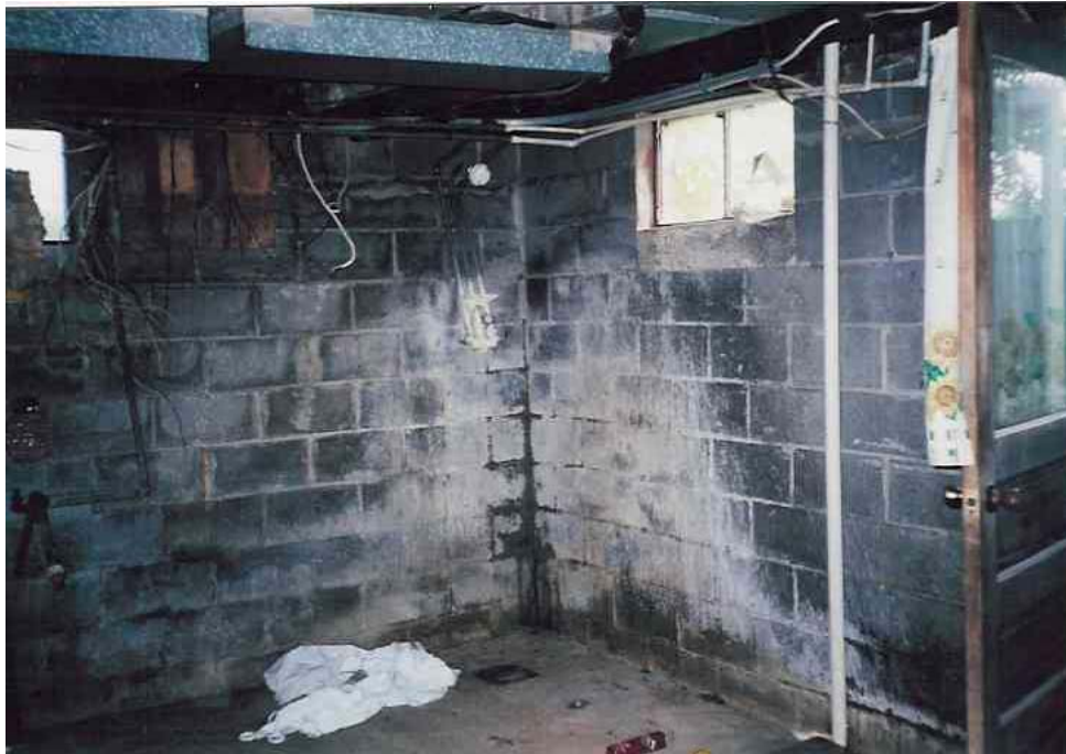
Figure 6.4 Basement walls of Indiana house 2
