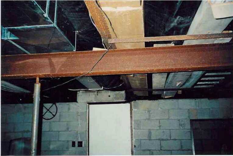
(a) Central ceiling beam spanning in the radial direction
