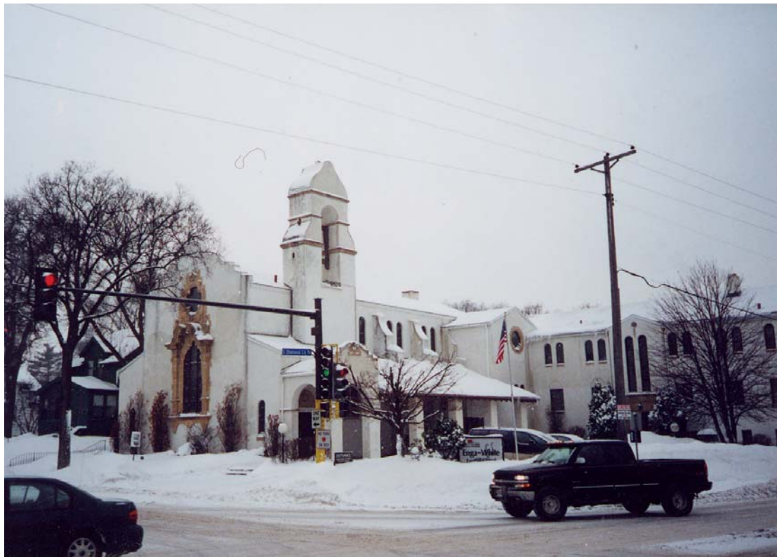
Figure 8.1 Stucco and tile block chapel
