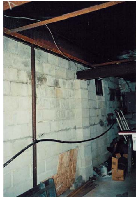
(b) Steel floor joists in transverse direction
